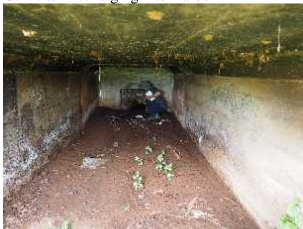
Substantial Sediment Deposition in Culvert
