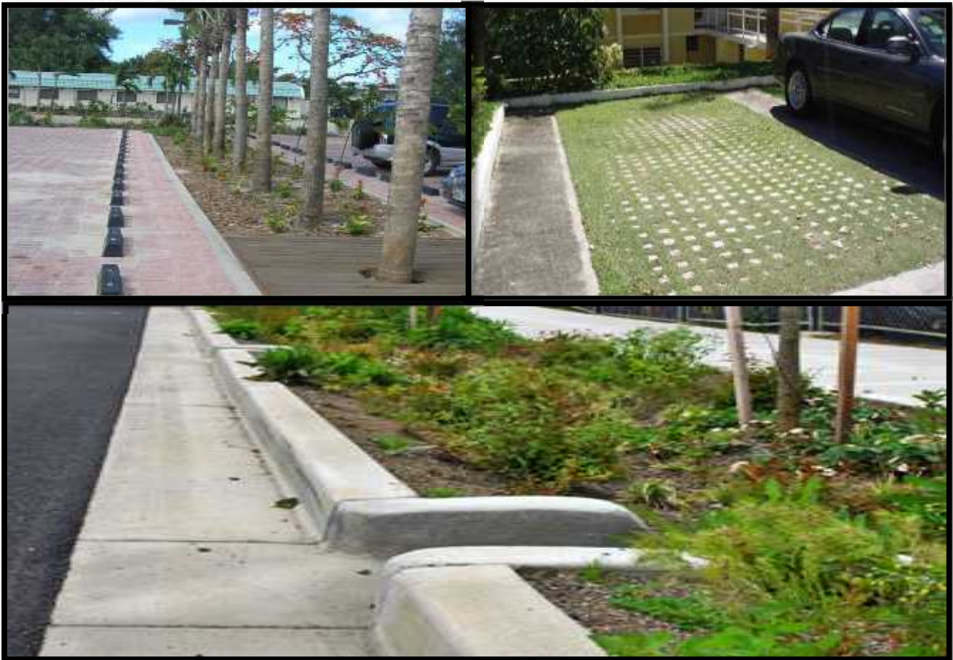
Figure 32. Examples of Low Impact Design (LID) Stormwater Treatment in Parking Lots
