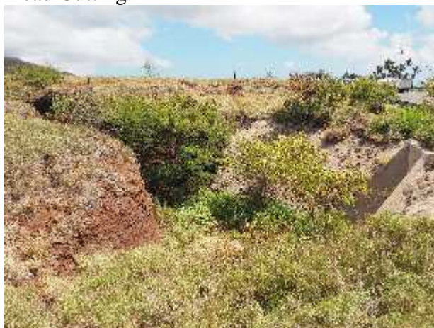
Culvert Backwall and Head Cutting
