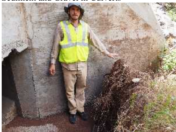
Extent of Vegetation at Entrance to Culvert Section 2 Mid-Level Agricultural Lands Waihe'e Makai Ditch:
