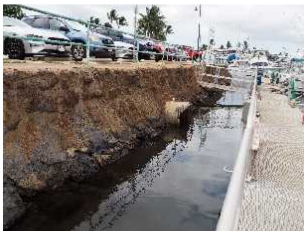
Culverts Discharging into Harbor
