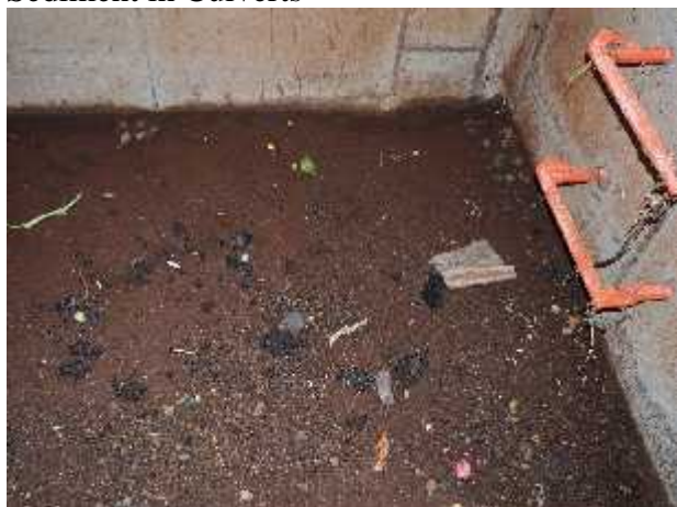
Sediment and Gravel in Culverts
