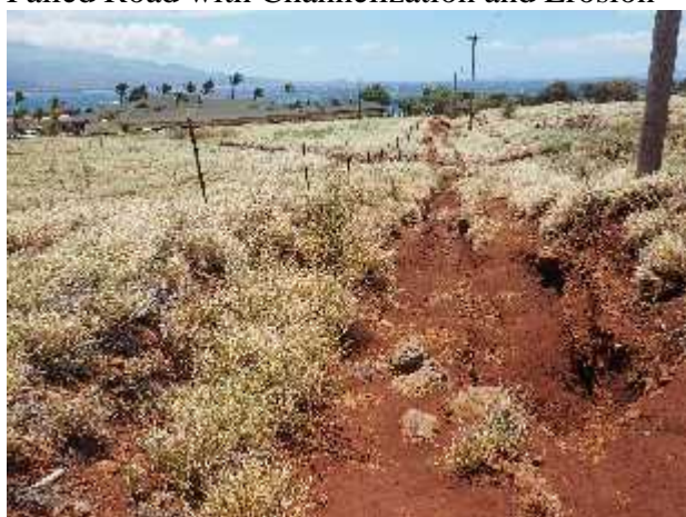
Failed Road with Channelization and Erosion Section 2 Mid-Level Agricultural Lands
