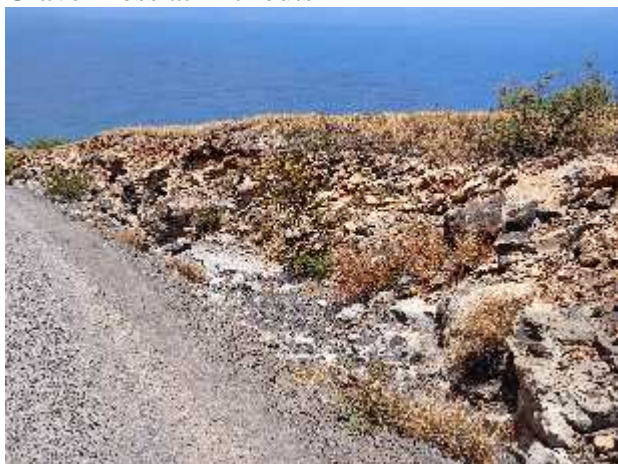
Channelization and Gravel Loss in Swale Section 1 Conservation Lands
