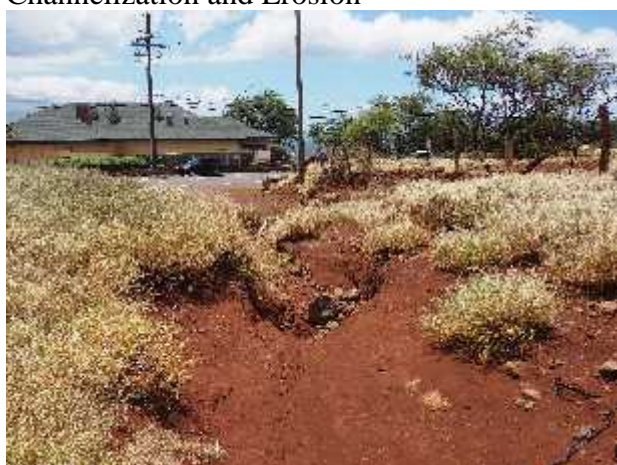
Failed Road with Channelization and Erosion
