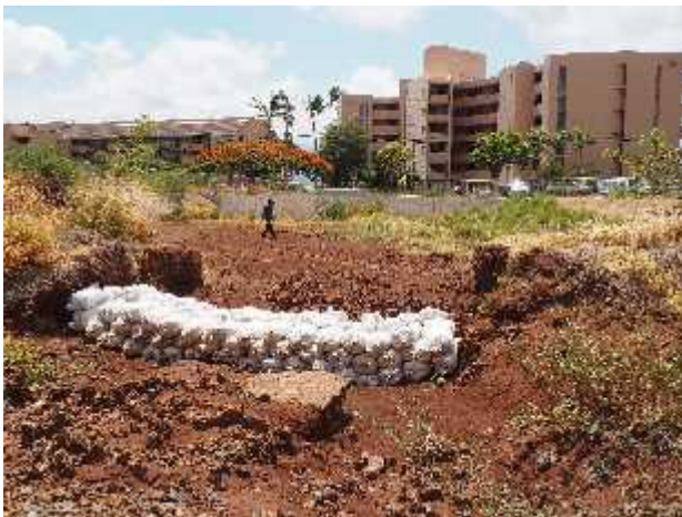
Sand Bags at Failed Control Structure
