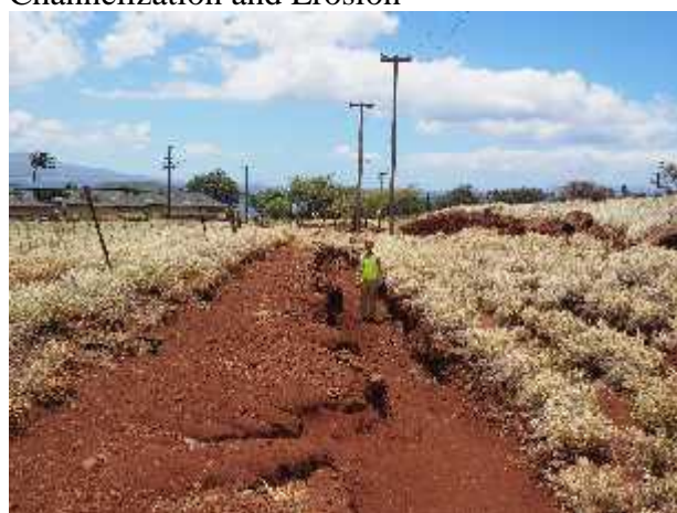
Failed Road with Channelization and Erosion
