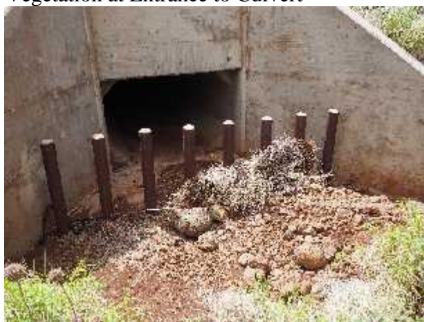
Sediment and Gravel at Culvert Entrance
