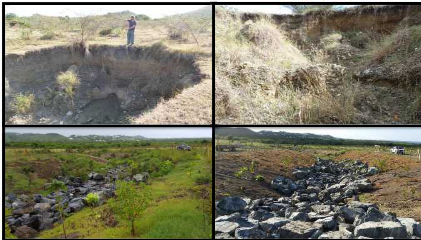
Figure 23. Examples of Head Cutting and Stabilization
