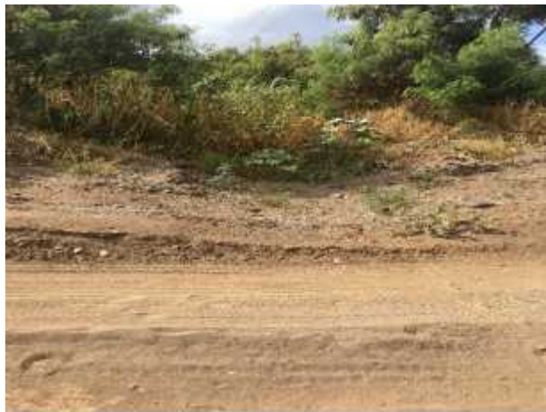
Road Crossing Pohakea Lacking BMPs
