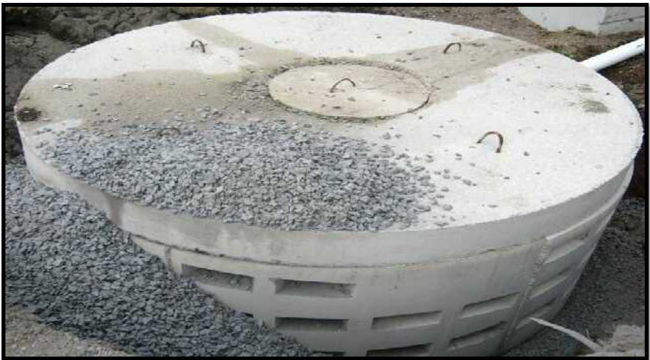
Figure 29. Stormwater Infiltration Well
