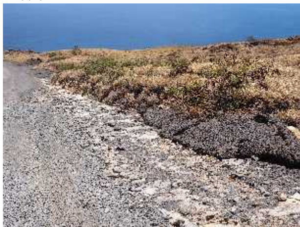
Gravel Loss in Swale
