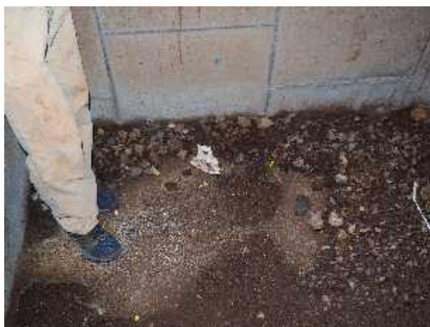
Sediment and Gravel in Culverts
