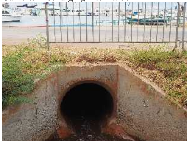
Culverts Discharging into Harbor
