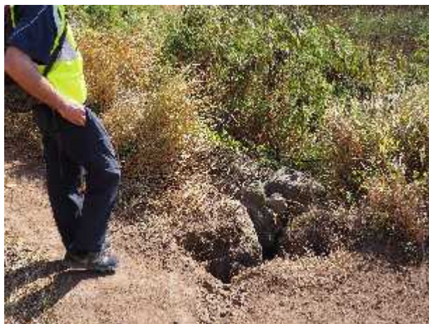
Erosion and Discharge from Road
