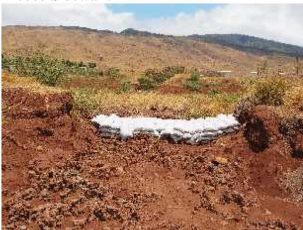
Failed Control Structure
