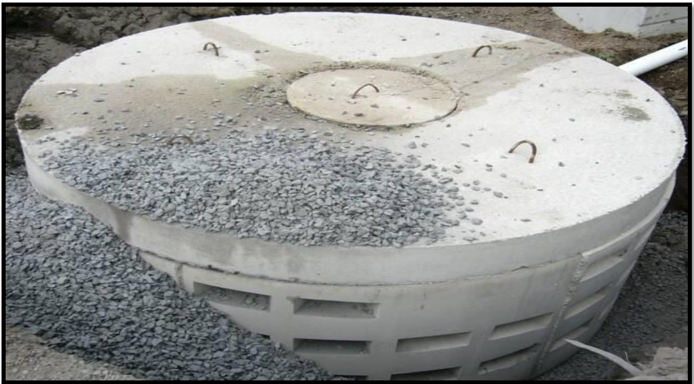
Figure 76. Stormwater Infiltration Well
