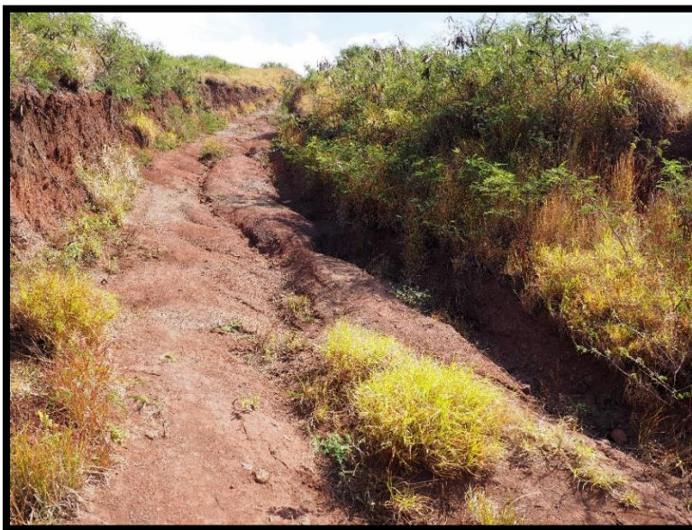
Figure 48. Example of Unmaintained Dirt Road
